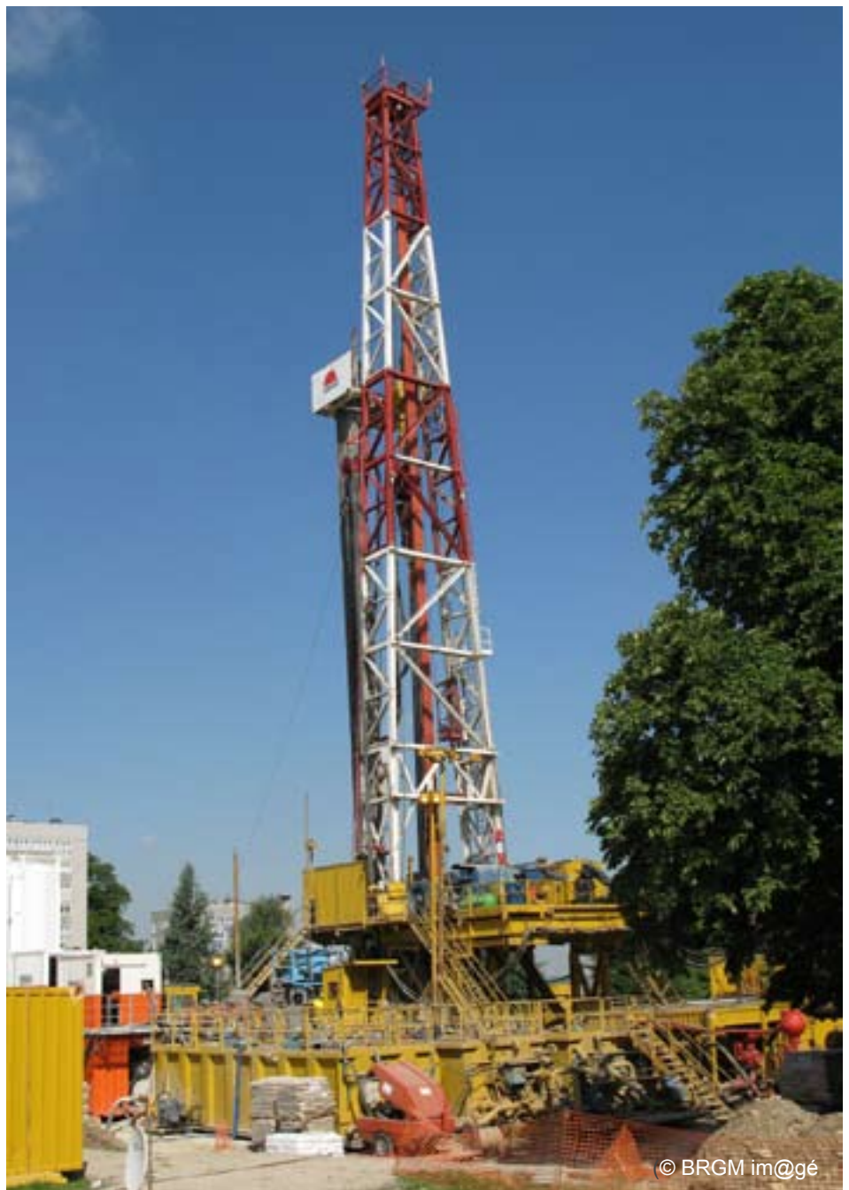
Drilling Rig for a new geothermal doublet in Sucy-en-Brie (Paris' area)
